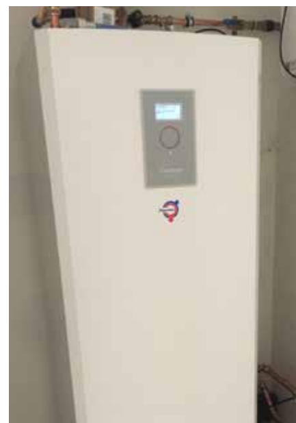
Thermia Comfort Optimum ground source heat pump
