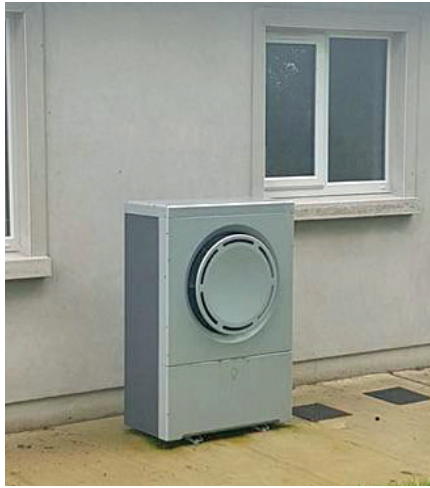
Thermia iTec 9 kW air source heat pump
