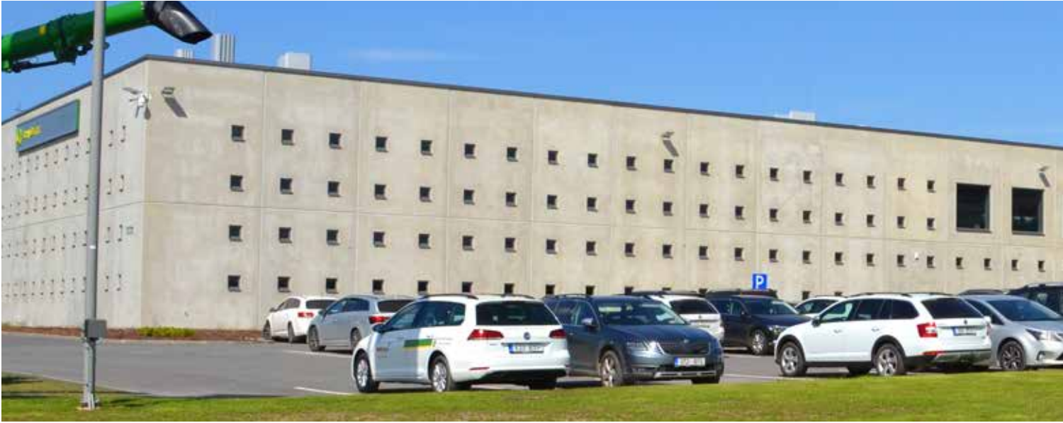
Baltic Agro Machinery headquarters in Estonia
