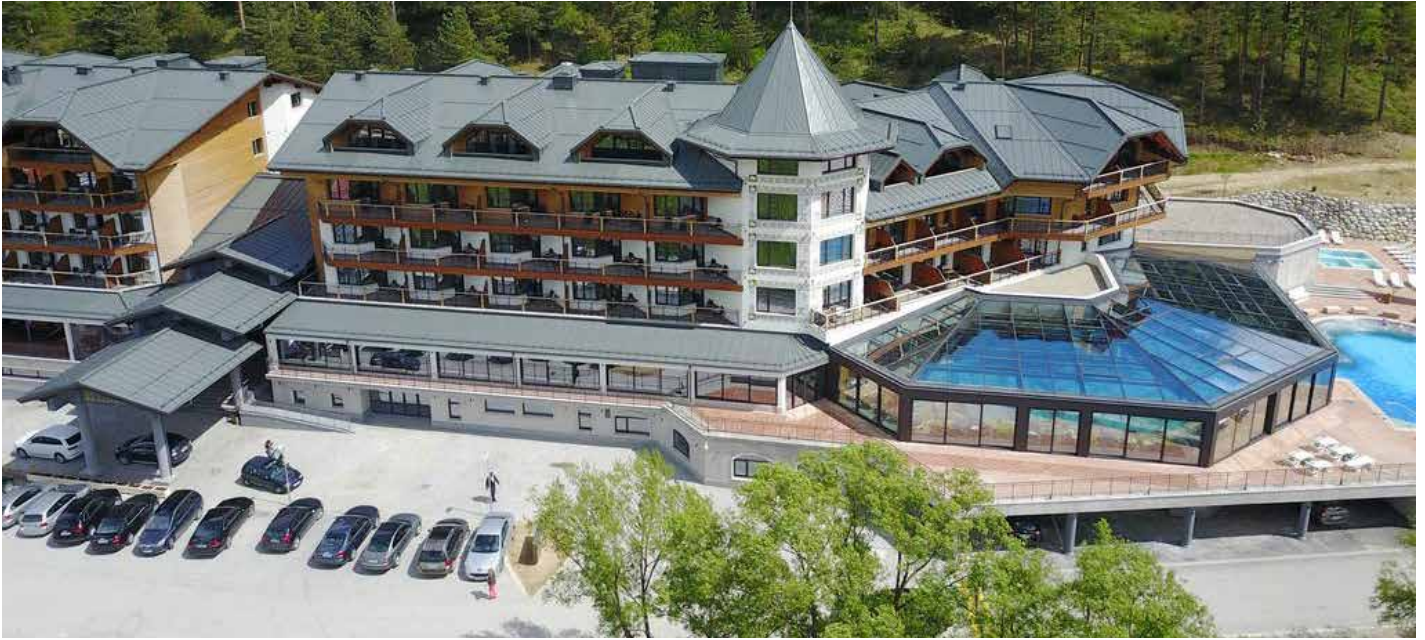
Hot Springs Medical & Spa - Front View
