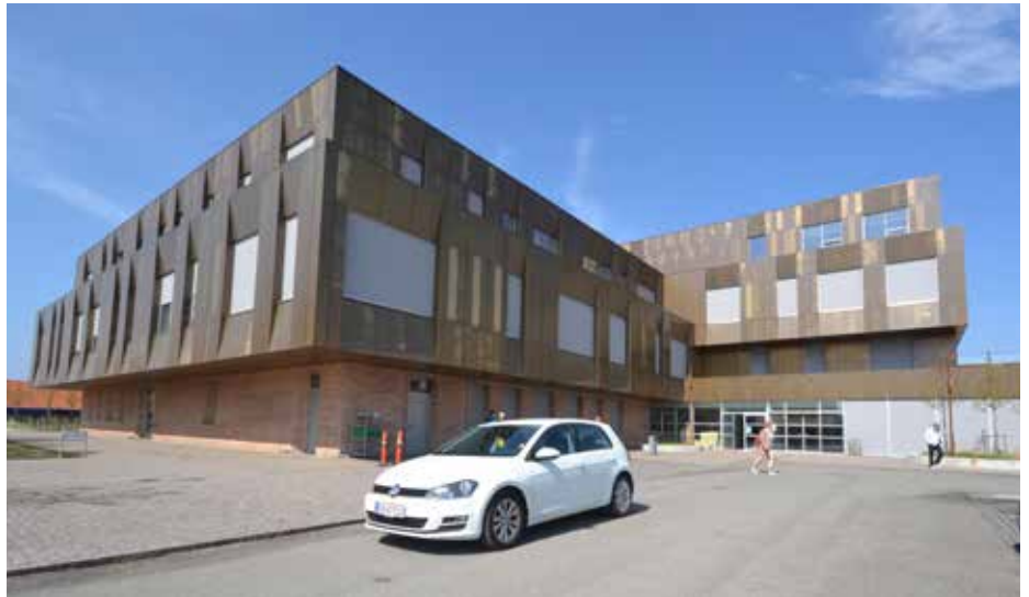
View of the Campus building from the parking area
