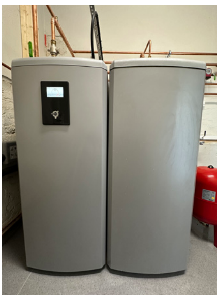
Thermia Athena Total Compact - indoor unit with WT-V 200 buffer tank Thermia Atlas with MBH – ground source heat pump with hot water tank
