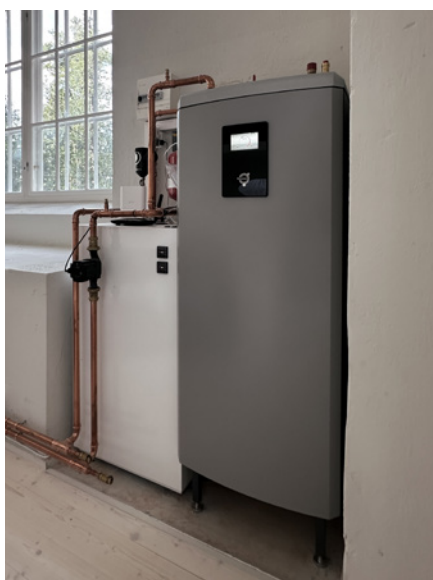
Thermia Athena Total Compact - indoor unit with WT-V 200 buffer tank Thermia Atlas with MBH – ground source heat pump with hot water tank
