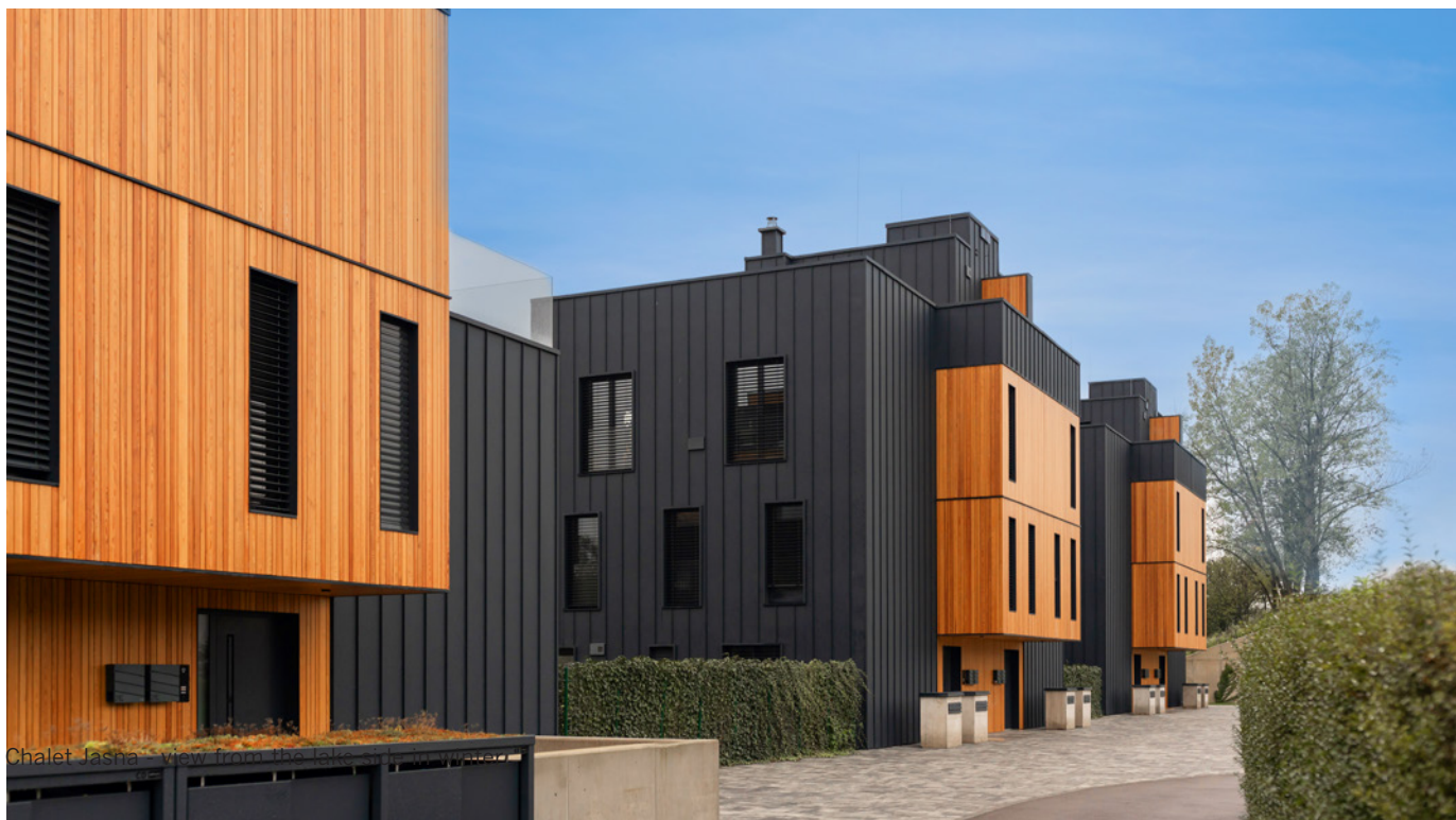
Apartment building "Zelena rašica"
